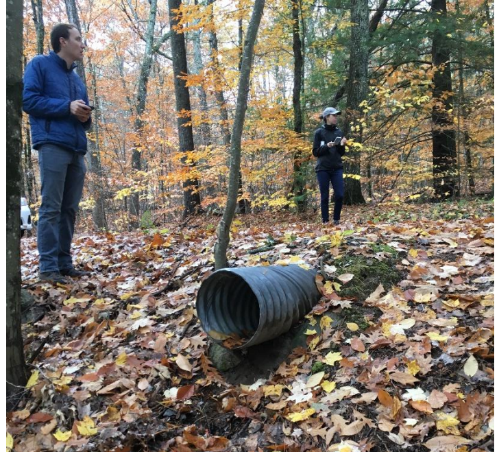
LEA and FBE staff document a perched culvert using handheld devices (above) and assess a lake public access point (below). Photo credit: FBE
