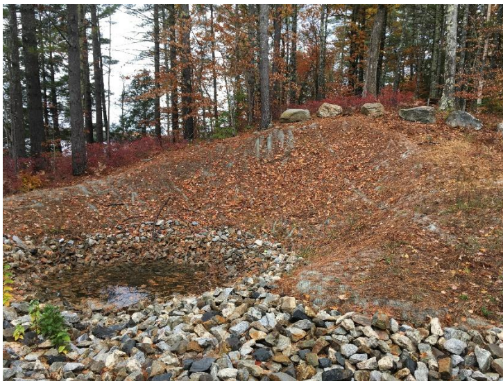
Examples of effective stormwater controls: catch basin and rip rap at the Trickey Pond public boat launch (left) and road shoulder armoring on Trickey Pond Road (right). Photo credit: FBE
