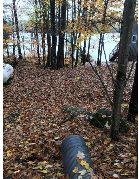
Culvert inlet (not visible among debris) (left) and perched culvert outlet (right).
