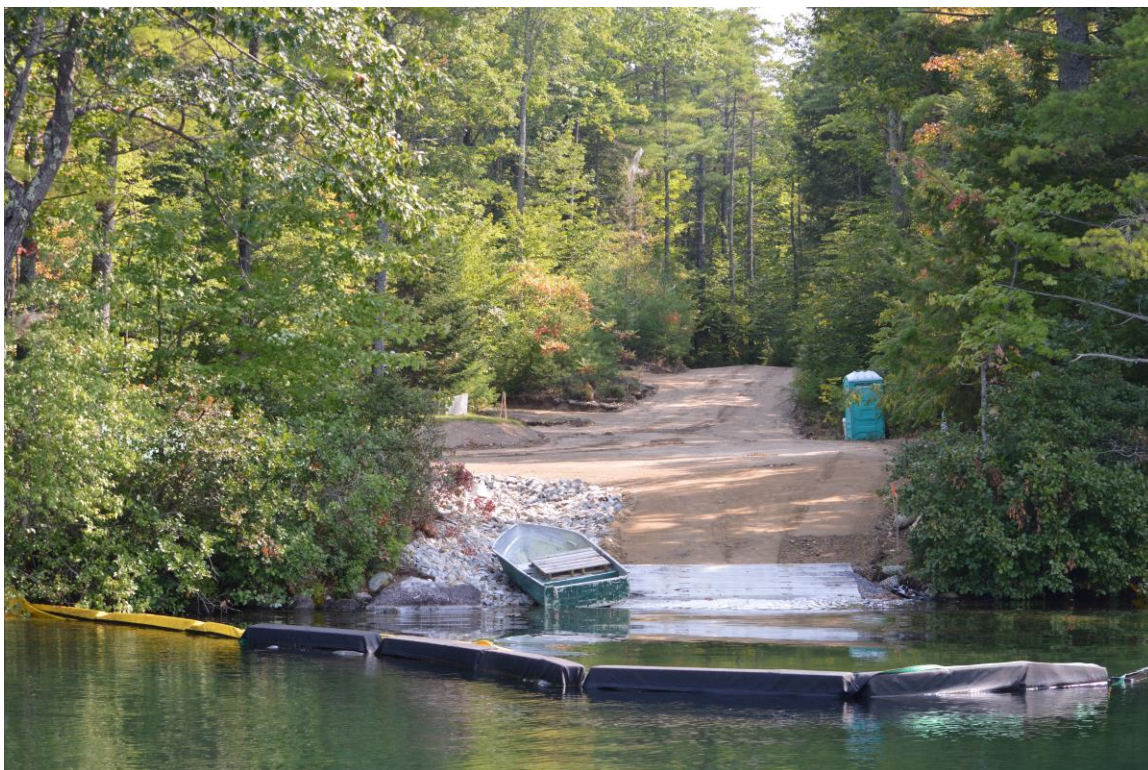
Picture shows the ramp toward the end of construction.
